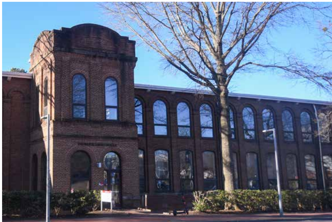
Tompkins Hall, pictured on Feb. 18, is home to the department of English at NC State. The building is located on north campus at 2211 Hillsborough Street.
